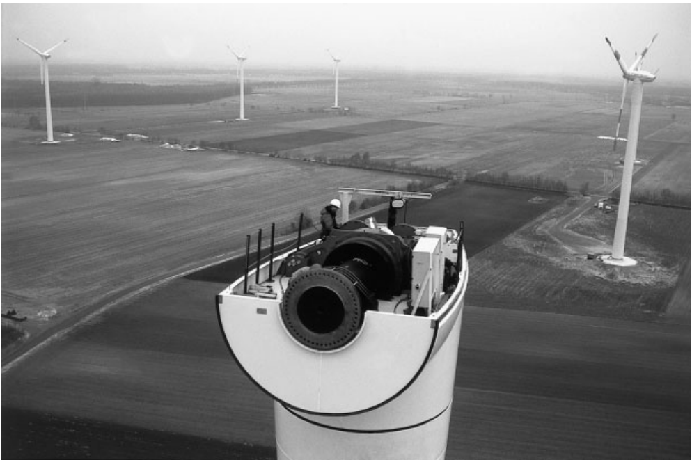
Figure 6.18 Turbine Assembly in the Air (1). (View of nacelle of 1.5 MW NEG Micon turbine after installation of low-speed shaft (front) and gearbox. The ring of bolt holes in the low-speed shaft flange for hub mountings are clearly visible). (Reproduced by permission of NEG Micon)
